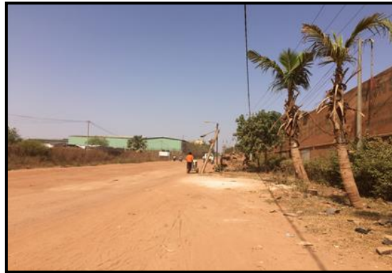
Picture 4: Off the main highway is an industrial area, but all the roads are unpaved
