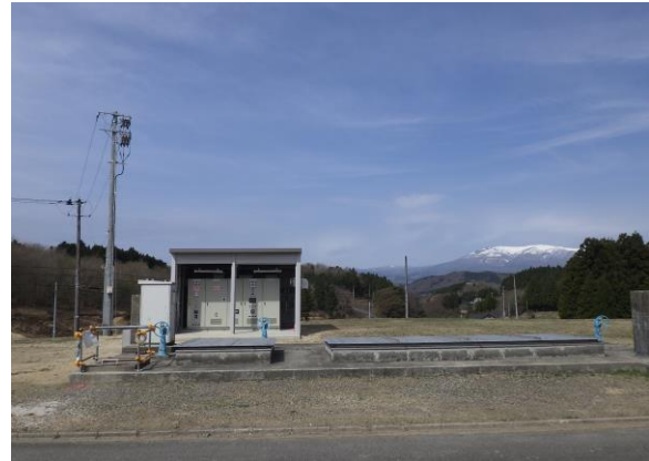
Building of an interconnection board
