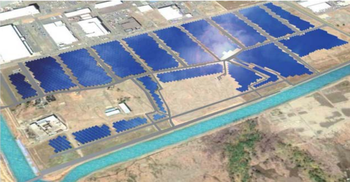
【CG Image of the completed Iwanuma-Rinku mega-solar power plant】
