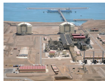
Natural gas liquefaction project in Peru
