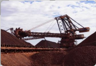
Roy Hill Iron Mine
