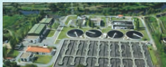
Water and wastewater treatment facility (Portugal)
