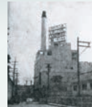
Unit No.1 at Manila Electric Company (Philippines)
