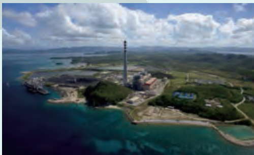
Pagbilao coal-fired power plant (Philippines)
