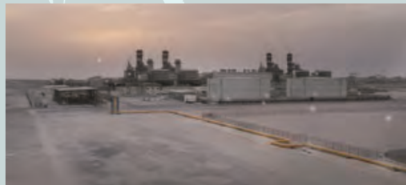
Power generation and desalination facilities of Shuweihat S2, which commenced operation in 2011 (UAE)
