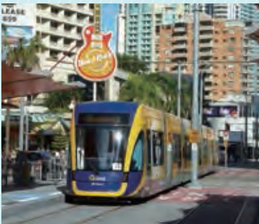
Light rail public transportation system building, operation, and maintenance project in Gold Coast (Australia)
