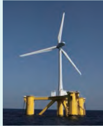
Turbine at Fukushima FORWARD floating offshore wind farm demonstration project (Japan) Source: Fukushima Offshore Wind Consortium
