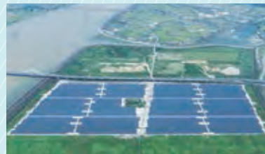
Kisozaki reclaimed land mega-solar project (Japan)
