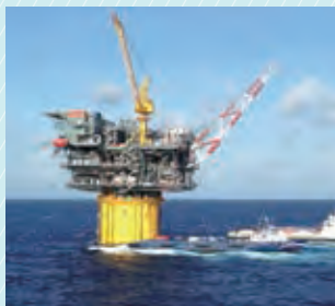
Spar-type floating oil and gas production and processing service platform operating in the Gulf of Mexico (U.S.)
