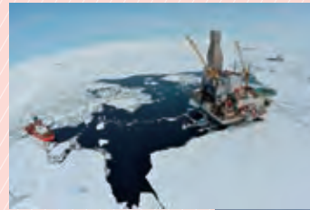
Sakhalin-1 Project (Russia)
