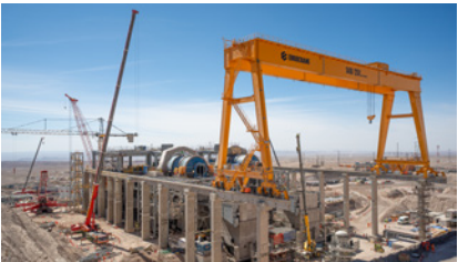
Chile: Centinela copper mine ball mill (under construction)
