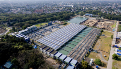
La Mesa Water Treatment Plant (Philippines)
