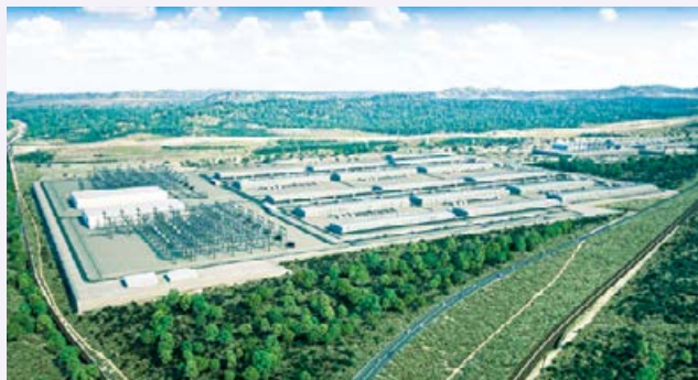
Image of hydrogen production site
