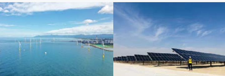
Courtesy of Akita Offshore Wind Corporation
