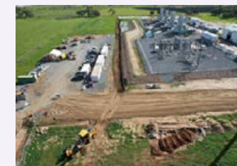
Demonstration facility under construction
