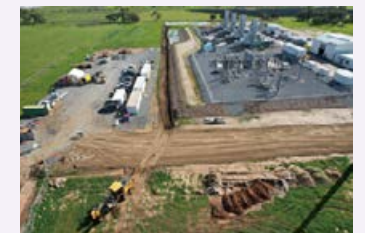
Demonstration facility under construction
