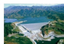
San Roque Hydroelectric Power Generation Project (Philippines)
