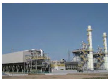
Nakasode Clean Power (Chiba Prefecture)
