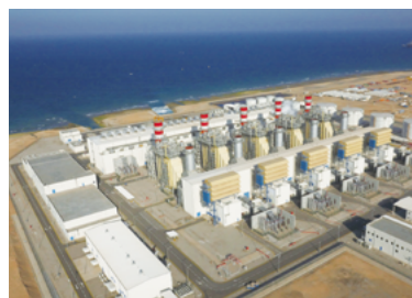
Power Generation Assets (Oman)
