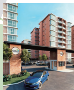
Sungai Long Residence (Malaysia)
