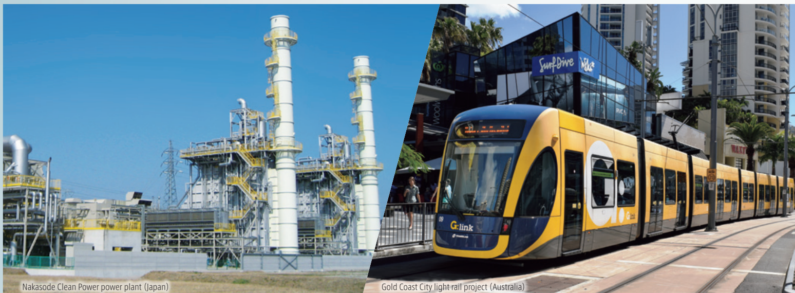
Nakasode Clean Power power plant (Japan)
