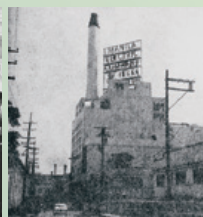
Manila Electric Company's generator No. 1 (Philippines)
