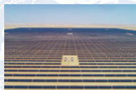
Amin Solar PV IPP Project (Oman)
