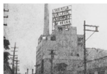
Manila Electric Company's generator No. 1 (Philippines)
