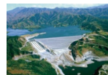
San Roque Hydroelectric Power Generation Project (Philippines)
