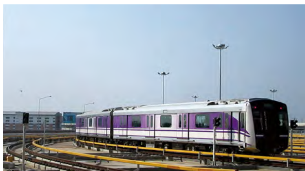
Rail System Supply for Purple Line Urban Railway in Bangkok (Thailand)
