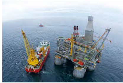
Sakhalin-1 Project (Russia)
