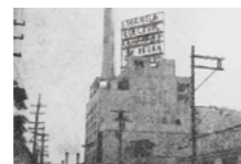
Manila Electric Company's generator No. 1 (Philippines)
