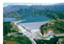
San Roque Hydroelectric Power Generation Project (Philippines)
