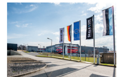
Skeleton production facility (Germany)
