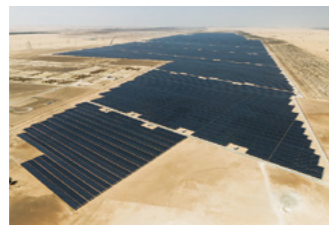
Sweihan Photovoltaic Independent Power Project
